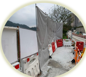
Temporary noise barriers installed at footpaths near Ma Yau Tong Village
